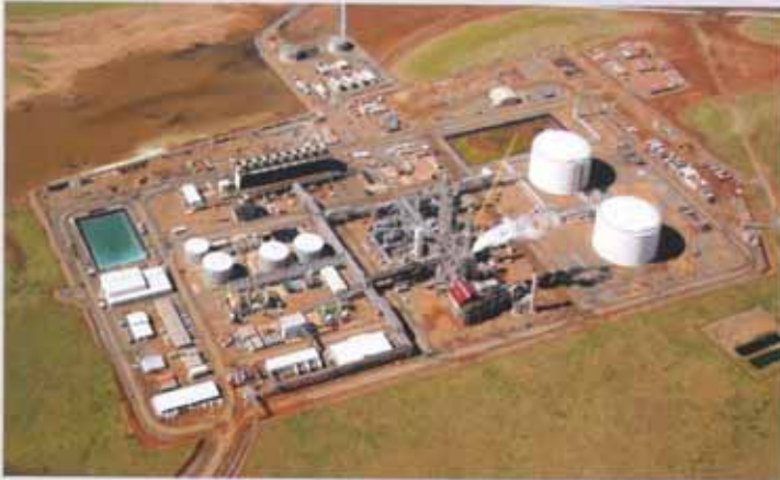
2200 MTPD Ammonia Plant at Australia World's the then largest single stream gas-based Ammonia Plant
