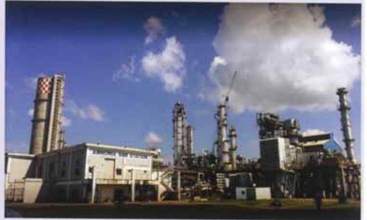
2200 MTPD Ammonia Plant at West Bengal World's First Coal bed Methane based Ammonia Plant
