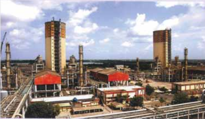
2*1890 MTPD Ammonia & 4*1662.5 MTPD Urea Plant at Gujarat Largest single location Urea Plant in India
