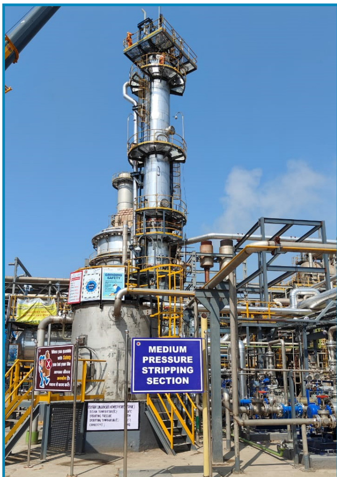
CFCL – EPCM Services for installation of Medium Pressure Stripper in Ammonia-I Plant at Gadepan
